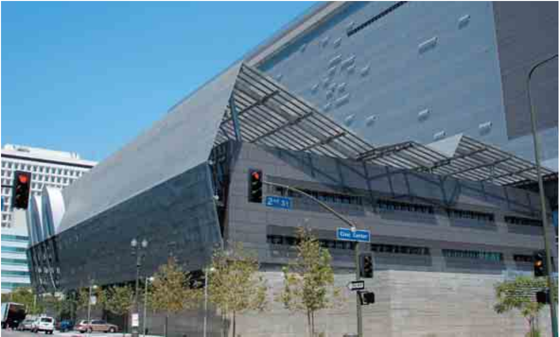
Los Angeles: Caltrans Station-district 7 headquarters door Morphosis (2004)
