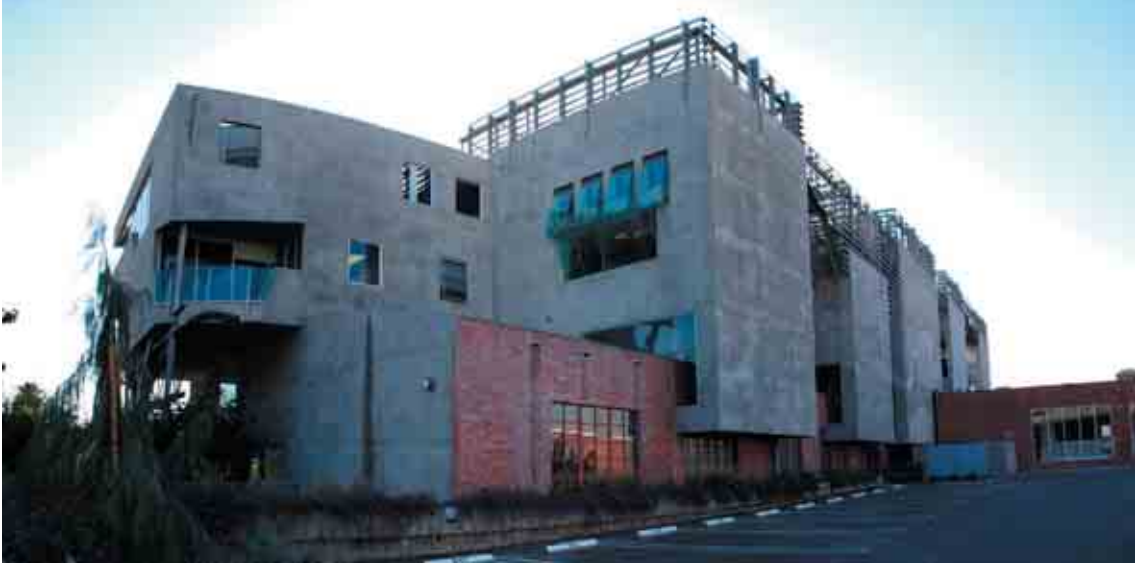
Los Angeles: Hayden residence in Culver City door Eric Owen Moss (1997)
